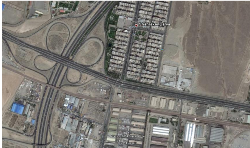
Figure 1. Interchange between Sattari Street and Azadegan highway.
